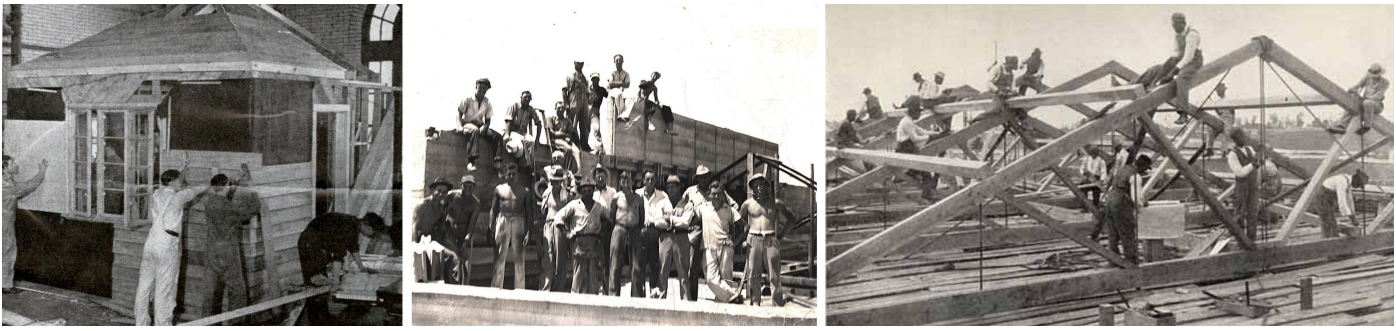
Figure 2. (a) Students at Carnegie Technical construct a demonstration house on campus, 1938, Source: Pittsburg Bulletin Index courtesy Carnegie Library of Pittsburgh; (b) Construction crew working on Anne Pfeiffer Chapel, circa 1938. Frank Lloyd Wright personally supervised the building of Pfeiffer Chapel, which was done in part by Florida Southern College students. Source: Special Collections, Florida Southern College Library, Lakeland, Florida. 21 (c) Students at Tuskegee Institute construct a building on their campus, early 1900s. Source: Library of Congress.
